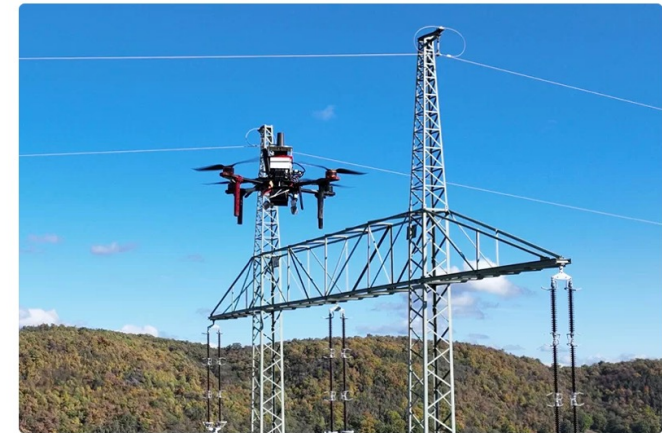
Drones can fly close to the power line and send real-time data to the operator interface.
